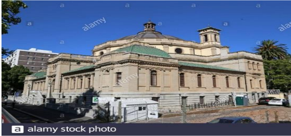
Figure 23: Centre for the Book, Cape Town, National Library of South Africa
